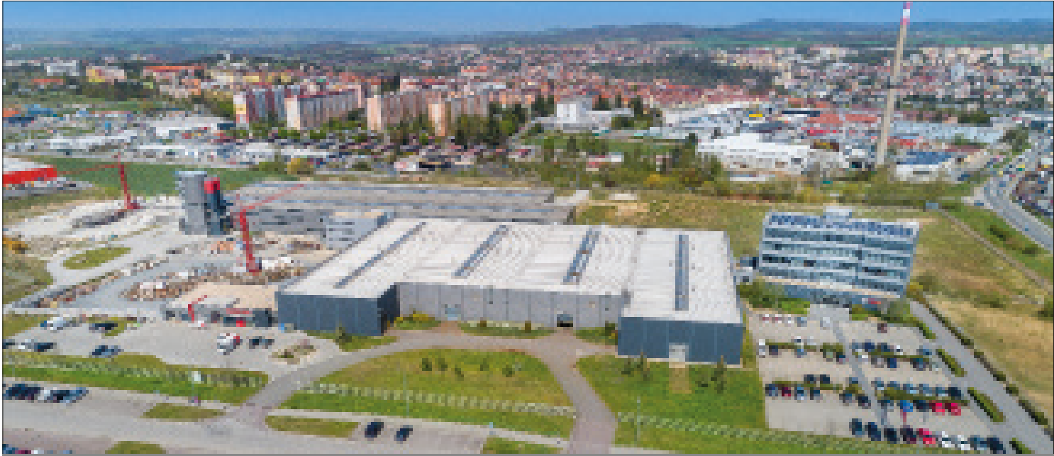
Company's headquarters and production halls
